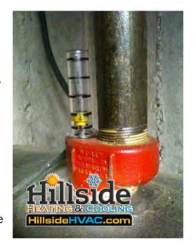
**Step 2:** Check the gauge or dipstick. Most tanks have a gauge or dipstick for checking the oil level. The meter typically features a dial or sliding indicator to display the current oil level, while the dipstick has a marker or line indicating the oil level.
